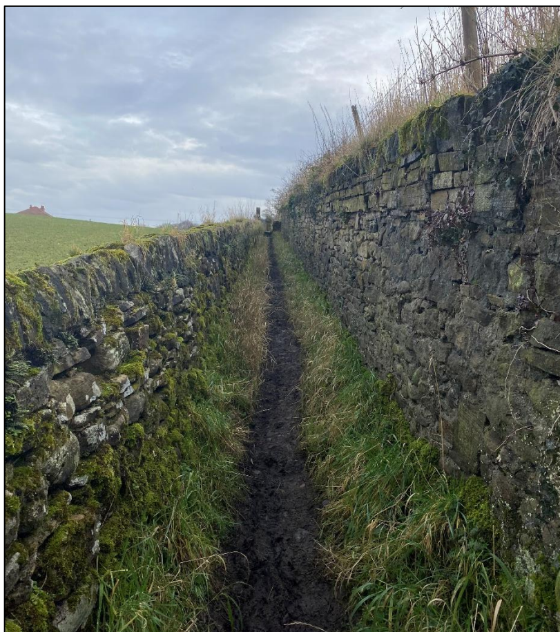
Site SH/027 Dry stone wall lined Public Right of Way Looking East
